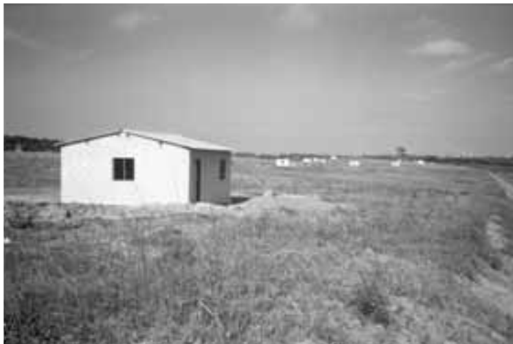
Above: A housing project in the Dukuduku forest after land has been cleared. This project was meant to lure people out of the forest: 2006
